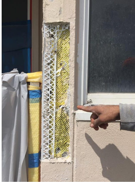
Picture 3: Area of stucco removed
