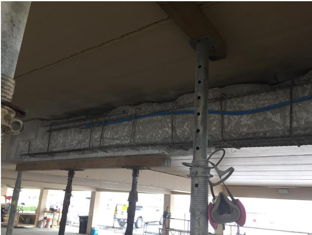
Picture 2: Inspected repair
