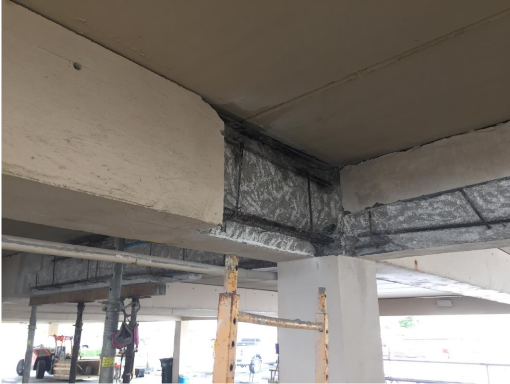
Picture 1: Inspected repair
